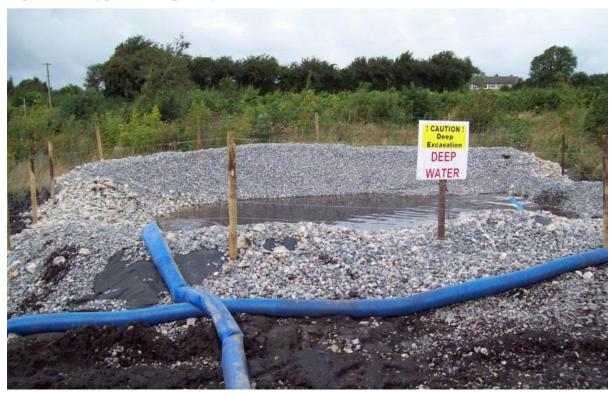
Figure 5.2: Typical Temporary Settlement Pond
